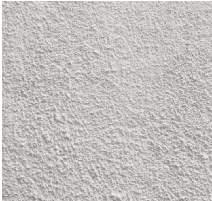
EIFS SIDING PAINTED IN PPG DELICATE WHITE 518-1
