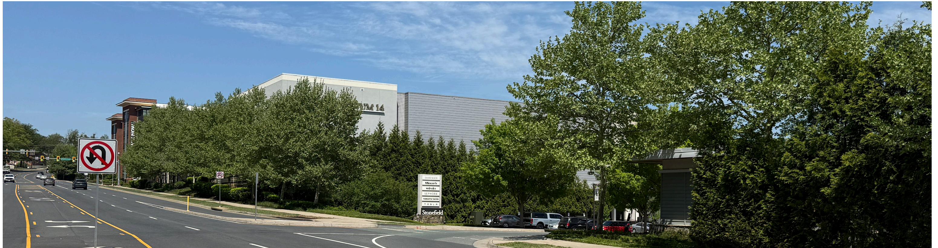
EXISTING APPROACH - NORTHBOUND HYDRAULIC ROAD
